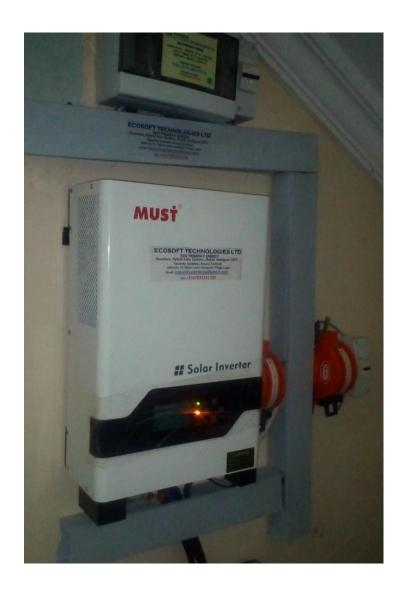
❖Installation of 5KVA 48V with 8 Units of 450 Watts Panels producing 3600 Watts of Solar Power for a client at Rukpokwu, Port Harcourt Rivers State, Nigeria. Completed by November 18, 2022.
