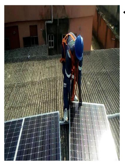
❖Installation of 5KVA 48V with 12 Units of 450 Watts Panels producing 5400 Watts of Solar Power for a client at No 20/22, Mojeed Omoledun Street, Ijegun Lagos Nigeria. Completed by November 26, 2022.
